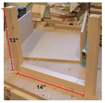
5. While your 1" x 4" boards dry, you can finish the leg construction. Cut your 2" x 2" board - (4) 13" long pieces and (2) 14" long pieces. Use RapidFuse to glue the pieces together as shown and clamp until dry.
